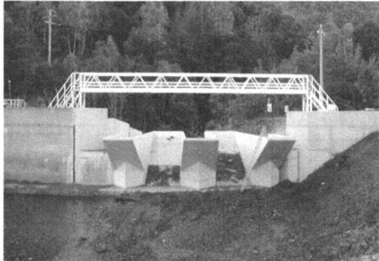
Figure 12. The piano keys weir (PK-Weir) carried out in 2006 to the Goulours dam (France).
